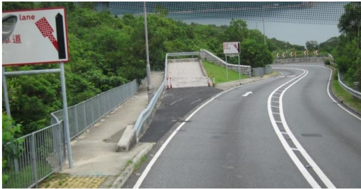
General View of the Arrester Bed for Southbound Traffic: Out-of-control vehicle is likely to overrun the facility and launched airborne into the forest
