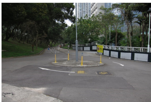
Lamp pole on the central island of a cycle track roundabout (left)
