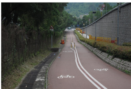
Protruded catchpit at the bottom of a long descent with a bend (right)
