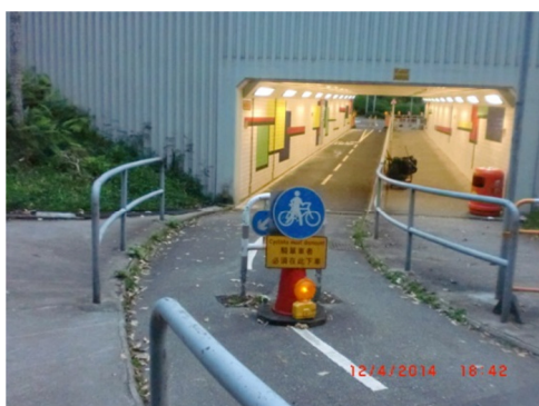
Headwall of a bicycle tunnel (left)
