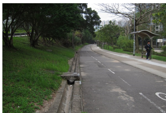
Protruded catchpit at the bottom of a long descent with a bend (right)
