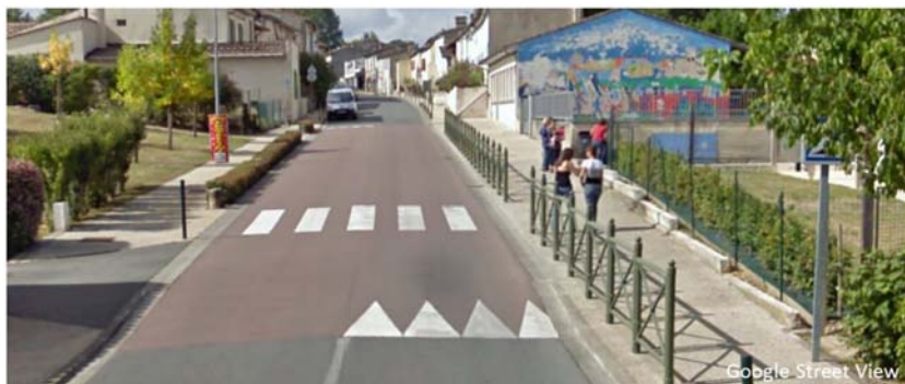
Diagram 4 Typical Raised Table with 7% Approach Ramps (L)
